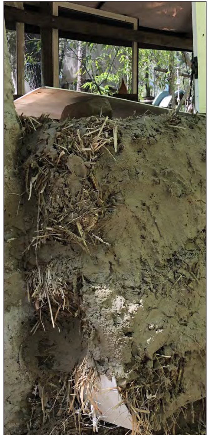
After stacking straw and wrapping in wire mesh the first layer of plastering begins (eg. with mud or cement)
