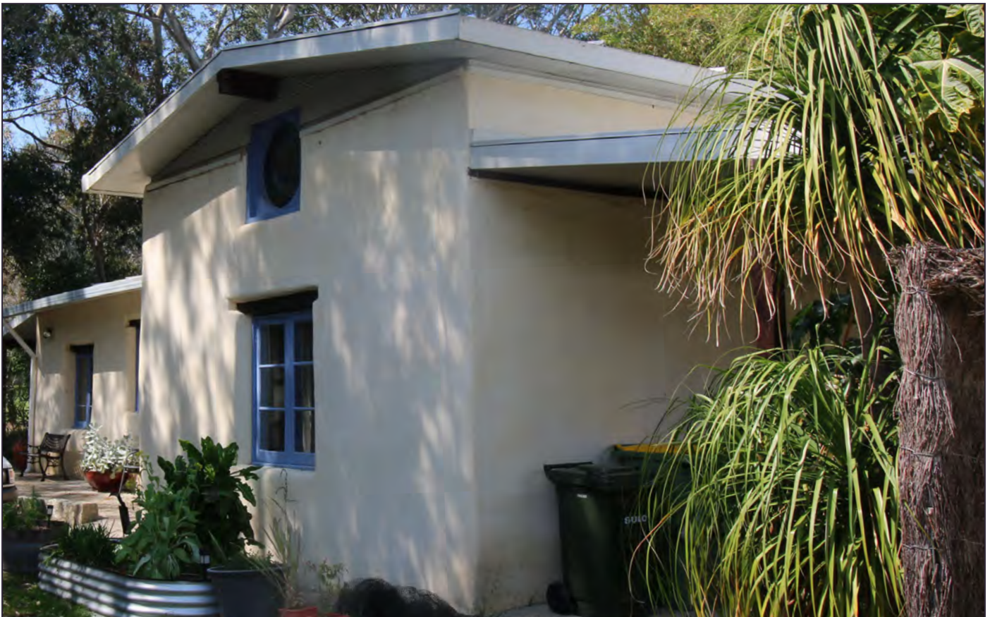
Cement render over straw bale construction
