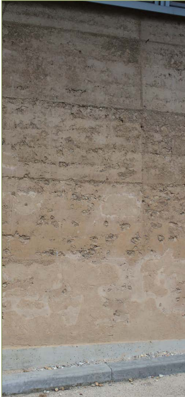
Rammed earth walls
