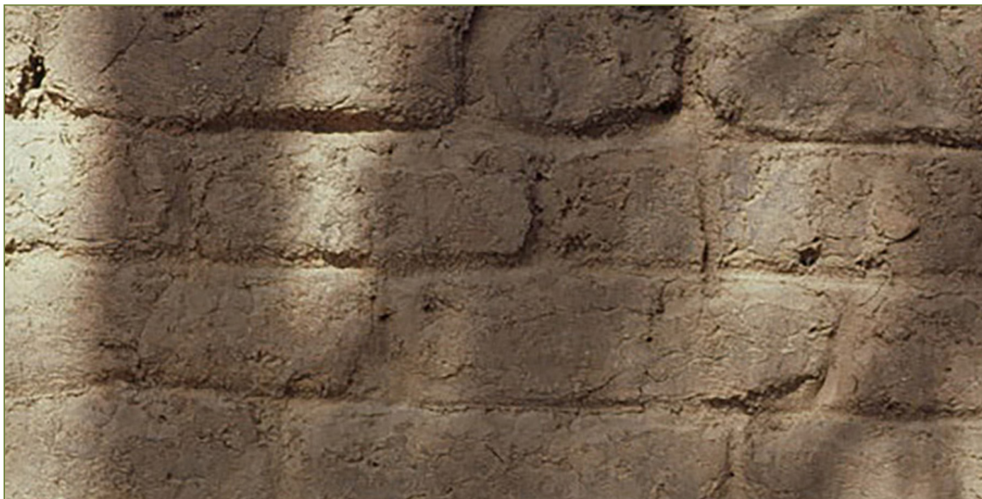
Mud brick wall
